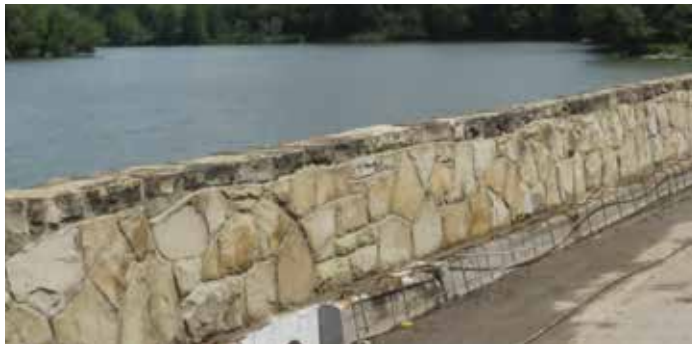
Pymatuning Dam PA - sandstone Heritage Restorer
