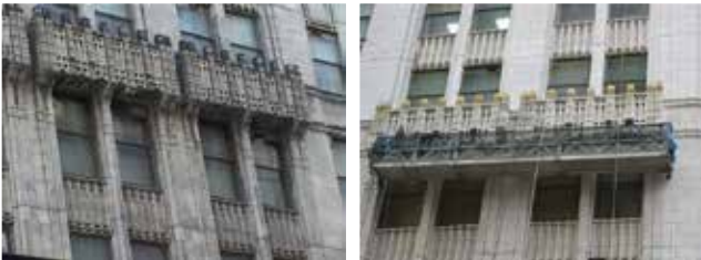
In the left photo shows the stark difference between cleaned and uncleaned. Inset is a close-up of the very heavy pollution stains.
