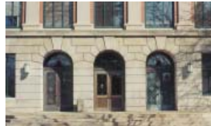
Limestone at Ohio State University's Administration building cleaned with Stripper Cream after a graffiti attack.
