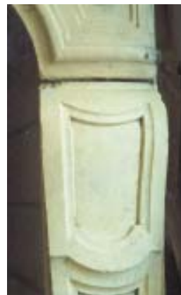
The same surround cleaned with SafeRestore by mason's apprentice. The job was done by hand and rinsed with a damp cloth.
