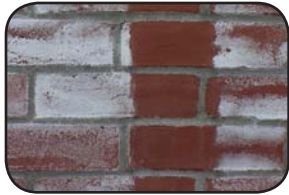
Efflorescence
