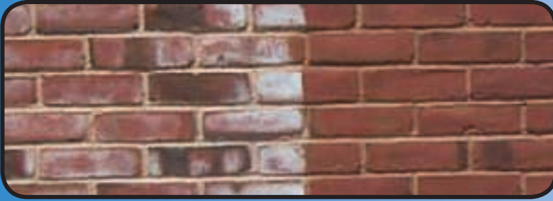
Efflorescence
