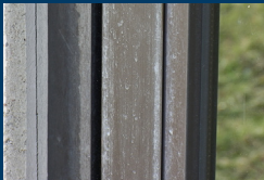
Before cleaning bronze anodized aluminum window frames
